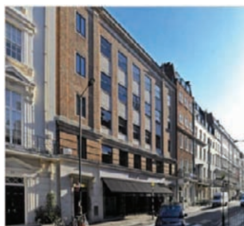
28-29 Dover Street, London W1
